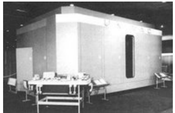
UNIVAC I, above, the first commercial electronic computer, achieved 1900 operations per second in a smaller and more efficient package than ENIAC.
